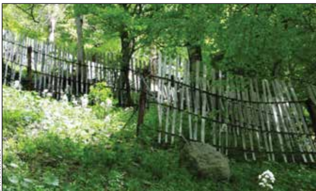
Deciduous forest as rockfall protection above the Arlberg Railway
