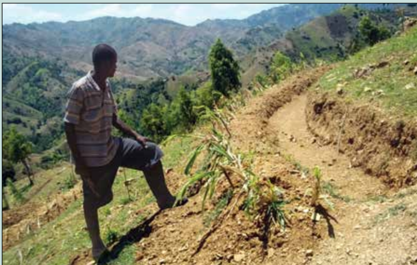
Construction of contour channels in the Canot watershed, 2012
