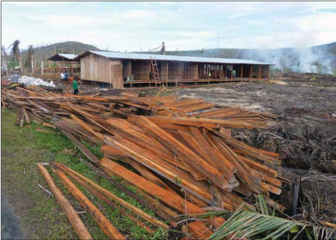
Temporary emergency housing constructed using coco lumber
